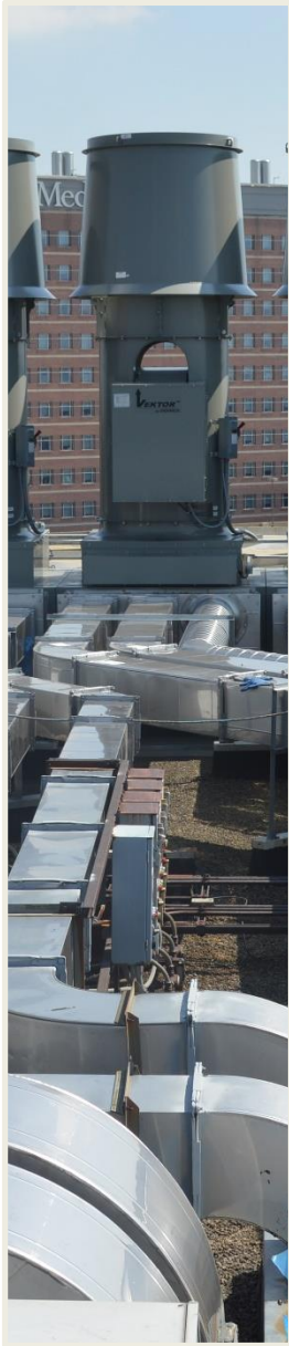
Philadelphia, VA Hospital Blood Lab Renovations
