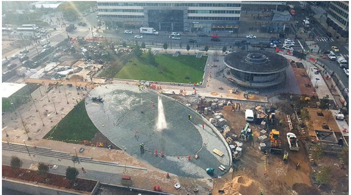
Love Park Iconic Fountain Piping, Plumbing, Trenching and Excavation (Philadelphia, PA)
